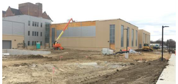
Grading Along Washington Blvd.
